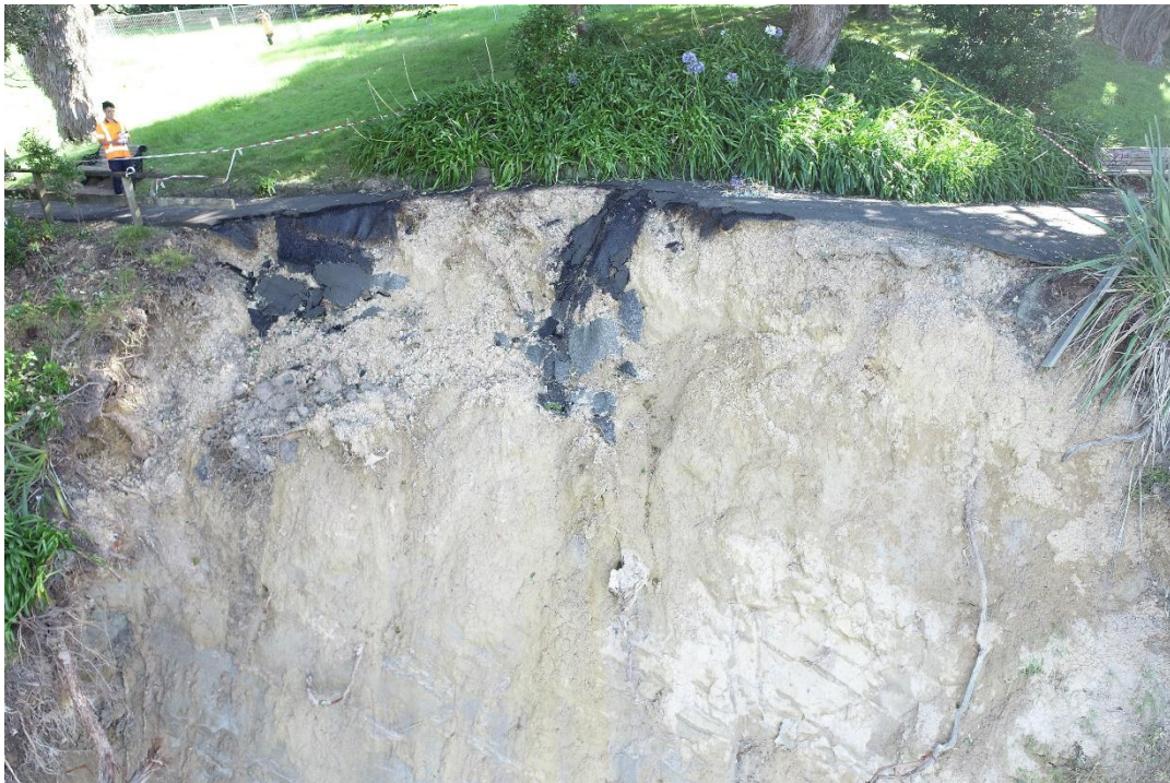
Slip 2 – Drone Footage showing exposed face
