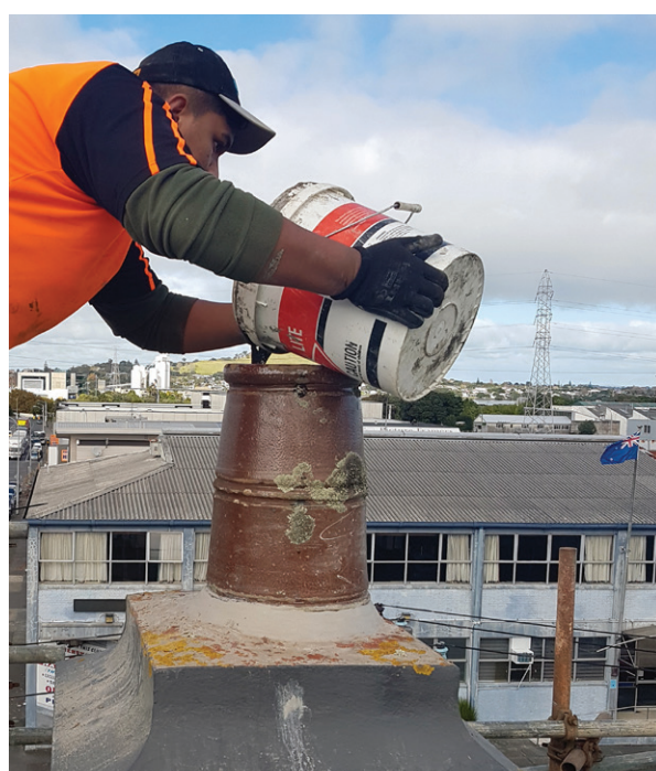
Builder pouring grout down the Post Office chimney. Photo: Anonymous.
