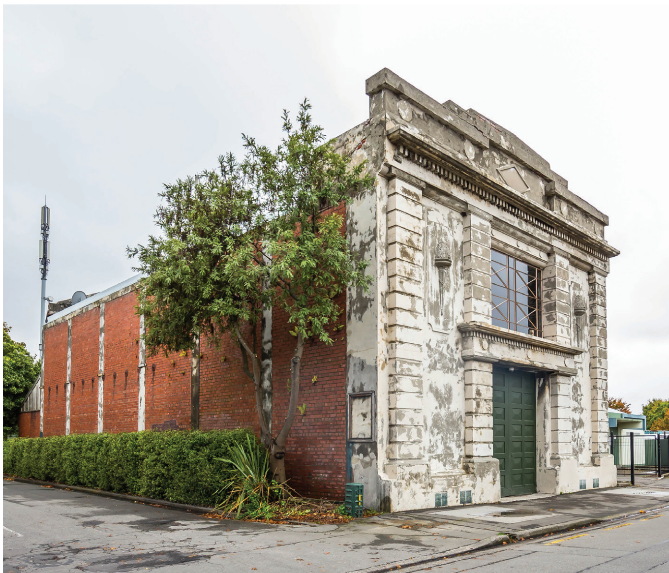
The Milton Street Substation, Sydenham, Christchurch. Photo: Clark Mauger.
